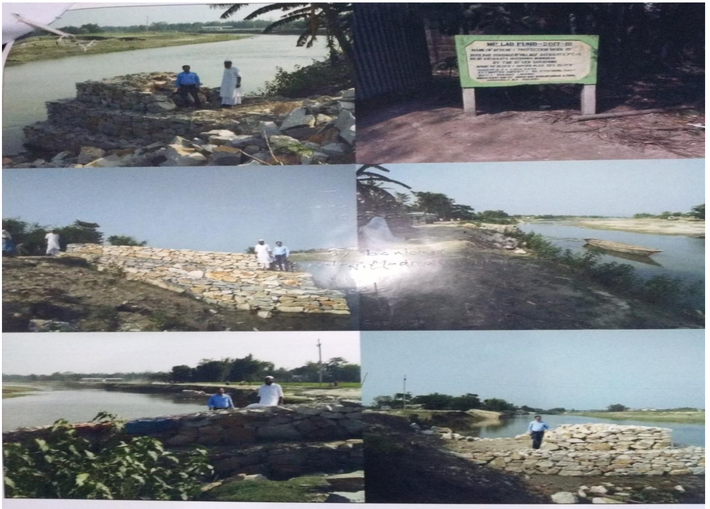
Protection work by Boulder Sausage at Vill. – Kazaikata Pt. – V near Kazaikata Madrassa by the river Gourang for the year 2016 -17 (Phase – I)
